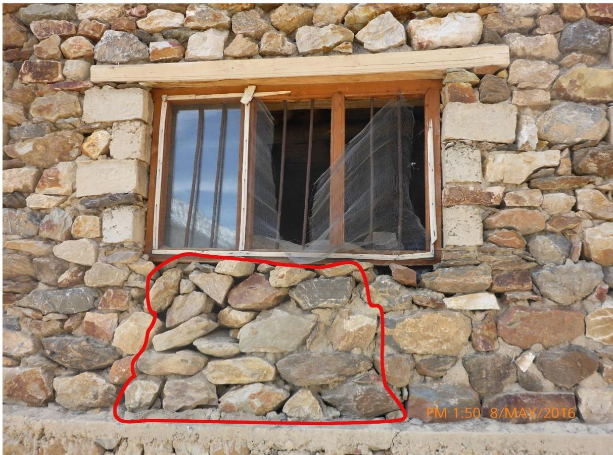
The repaired wall with the part removed by the bear highlighted
